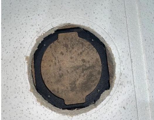
Complete your wiring of the fixture via the hole connect power and data to the Moonlite 80 and install and secure the Moonlite 80 with the 4 long screws to the retaining section.
